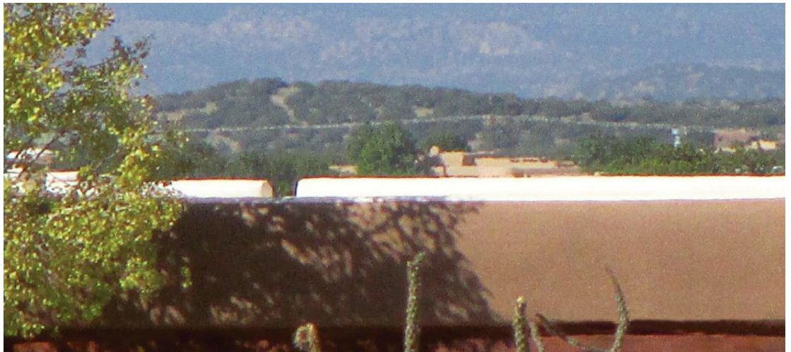
The strip of white on this roof shows how bright and reflective the bright white silicone appears on roofs.
